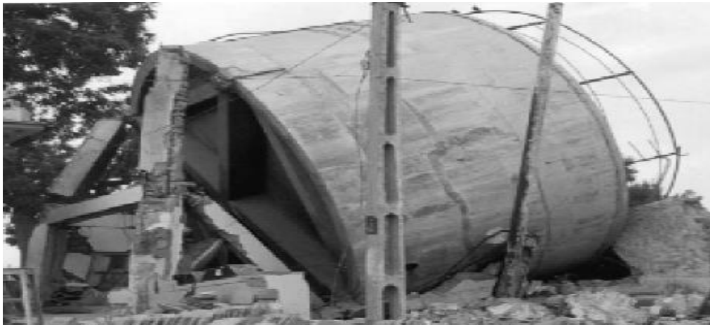
Figure 2 Collapsed water tank in Bhachau (Source: Rai, 2003)
