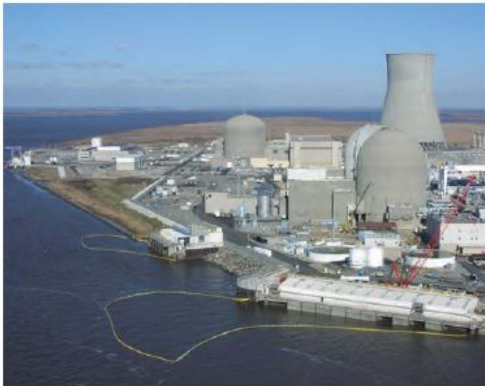
A shut down power plant
