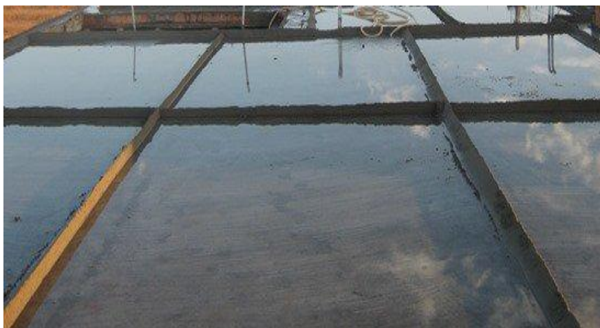
Fig 2: ponding curing
