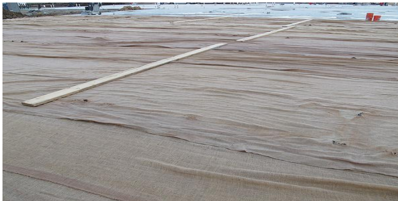
Fig 4: Wet curing
