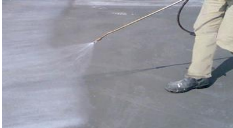
Fig3: Spraying or fogging curing
