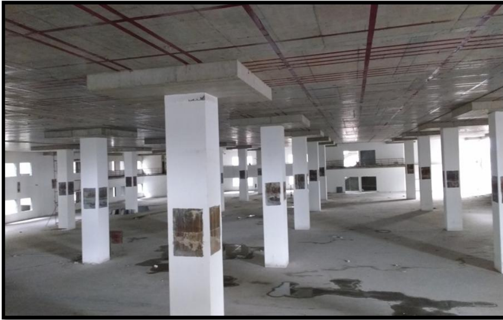
Figure 2: Flat Slab System with Drop
