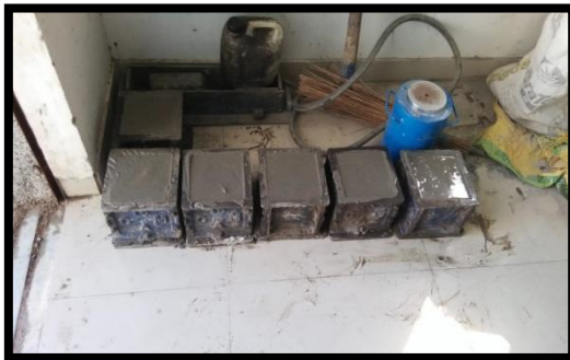
Figure: -2. Cube Casting
