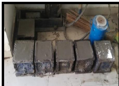
Figure: -5.Cube Casting
