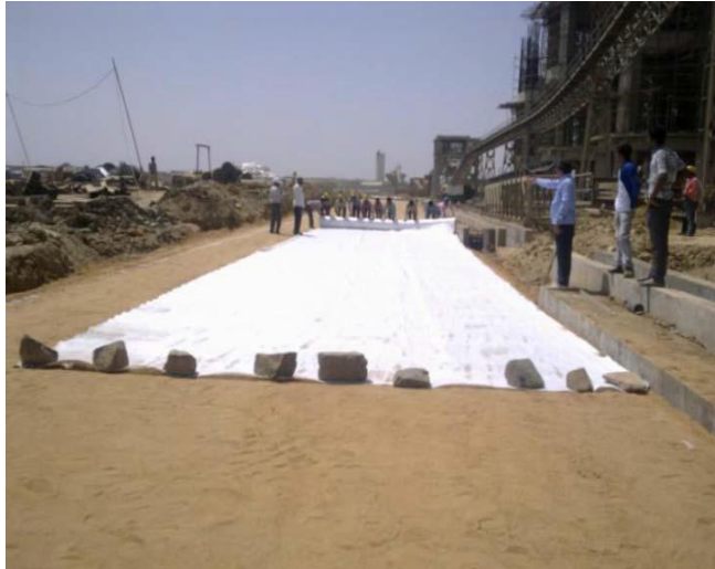
Fig. Laying of Non-woven Geotextile
