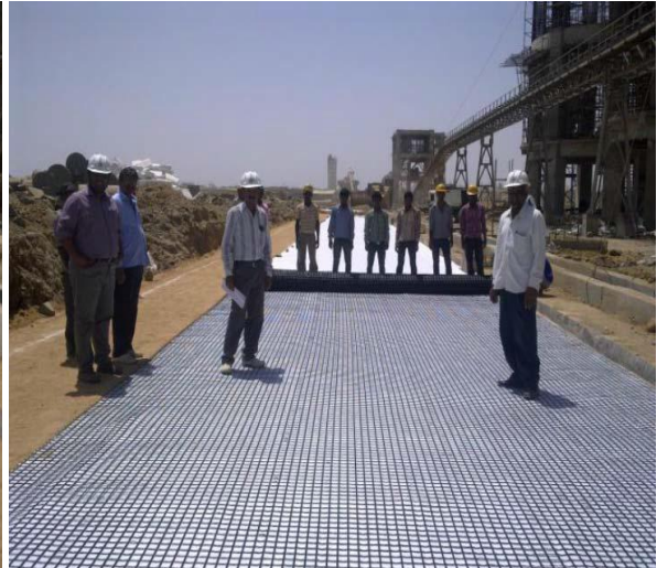
Fig. Laying of Geogrid
