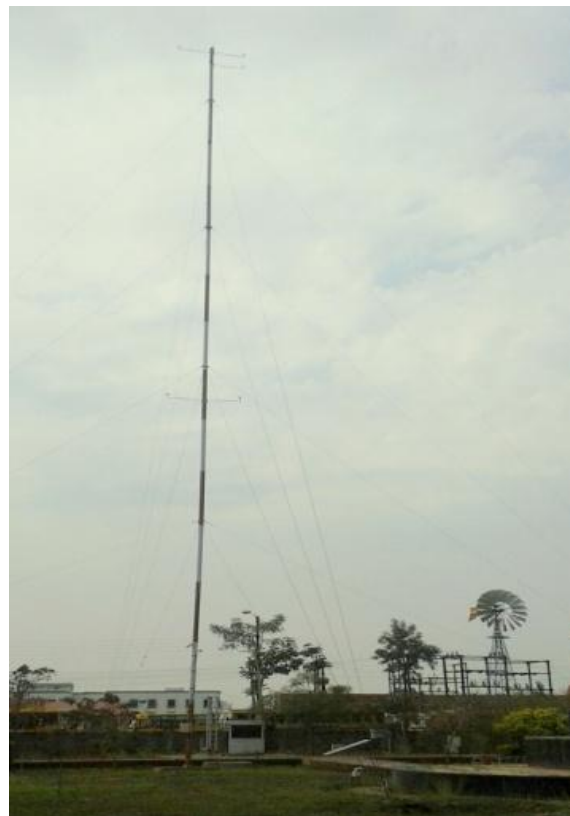
Fig. 4 Wind masts at energy park, RGPV
