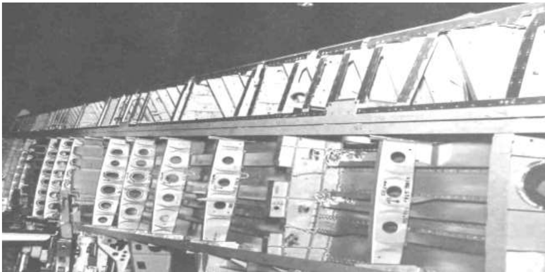
Figure 727 aircraft wing with lower skin not installed showing the wing rib
