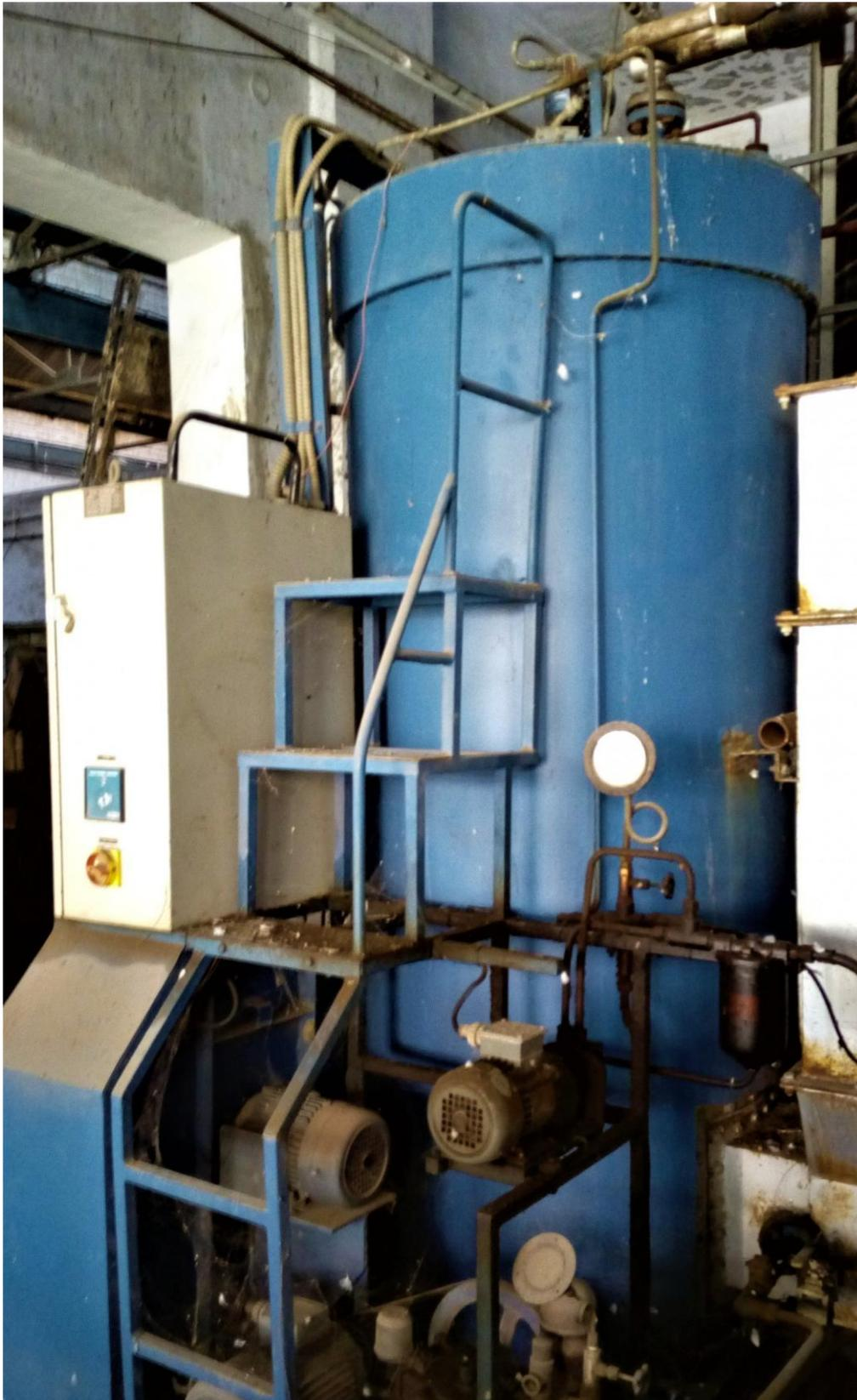
*Figure 3.1. Diesel fired boiler*
