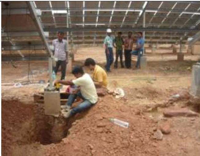
Photo 3 Sonic Integrity Testing at site
