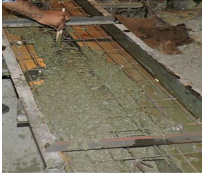
Figure 4. Pouring of concrete in girder form work
