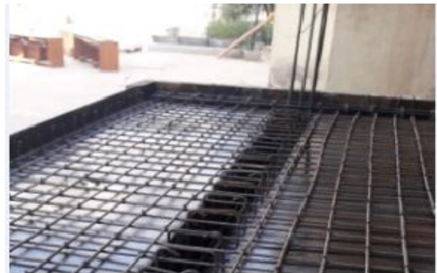
Figure 5: Reinforcement of beams, columns & slab
