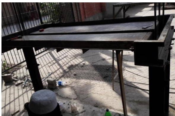
Figure 4: 1 st storey form-work
