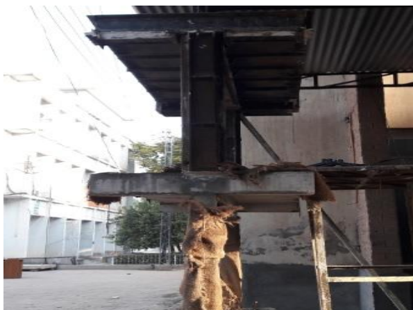
Figure 10: 2 nd storey form-work
