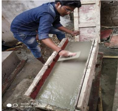
Fig.5- the casting of beam
