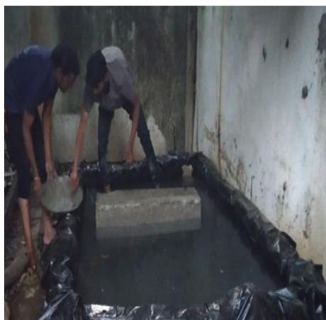
Fig.7-curing of beam
