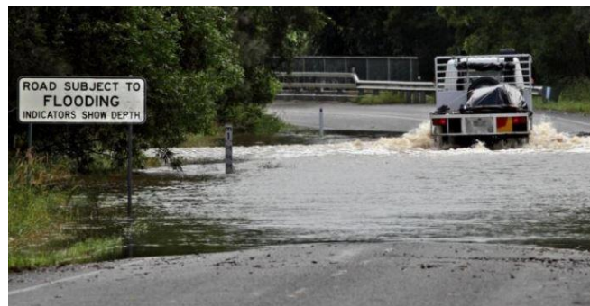
Fig. 2. Traditional road subject to flooding G9-21-1 sign.
