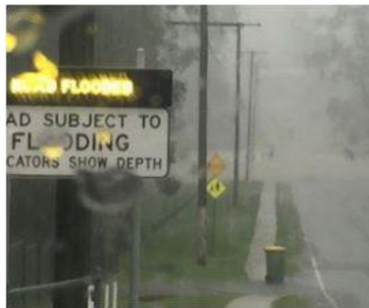
Fig. 4. LED 'ROAD FLOODED' text matrix board on G9-21-1 sign at the actual site [8].
