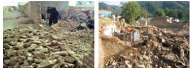
Figure 1.3. Typical damage caused by the Dalbandin Earthquake in 2011 [9]
