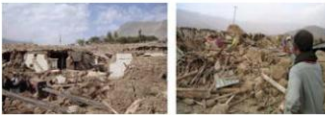
Figure 1.2. Total collapse of adobe houses during the Ziarat Earthquake in 2008 [9]
