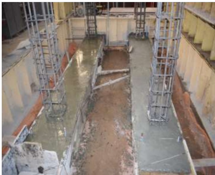
Figure 3: RC footing after concreting
