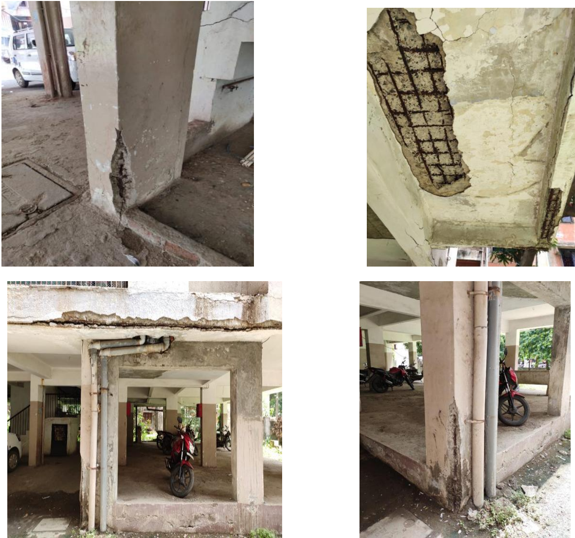
Figure 1 Deterioration of concrete in column, slab, beam
