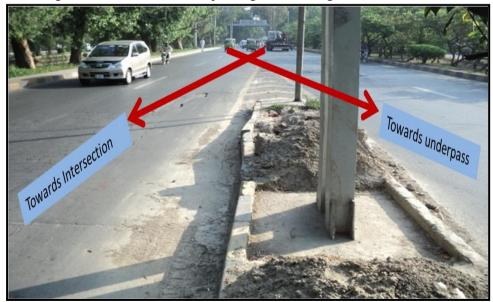
Figure 1. The deficient geometry at the Jail Road underpass creates unnecessary weaving and safety hazards
