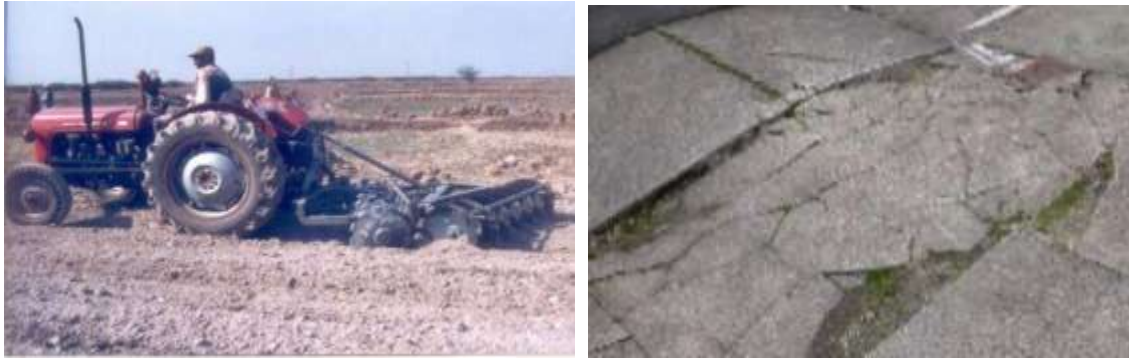
Figure 3: Fly ash mixing with a disc harrow and Road on Black Cotton Soil
