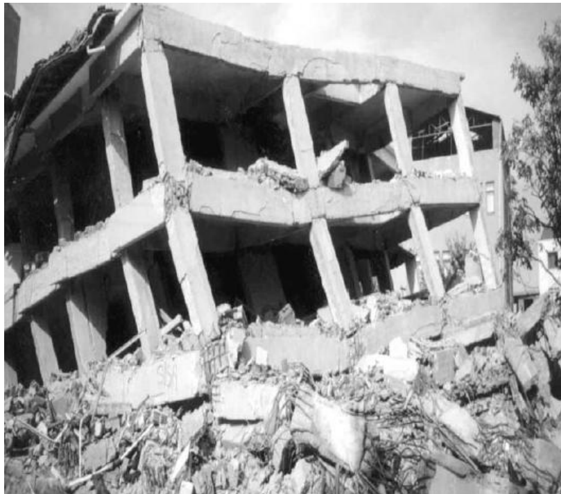
Figure 1. Failure of joint during Turkey earthquake, 1999
