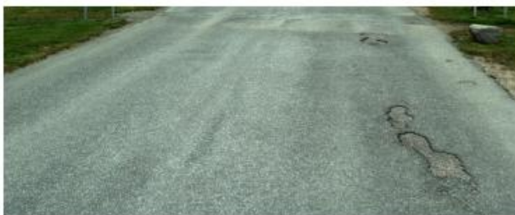
Figure 3: Potholes
