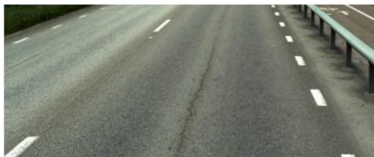
Figure 1: Longitudinal cracking
