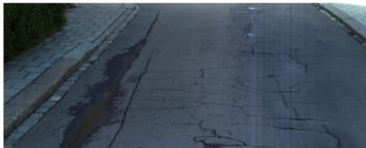
Figure 2: Fatigue cracking
