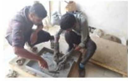
3. Mixing of brick mortar
