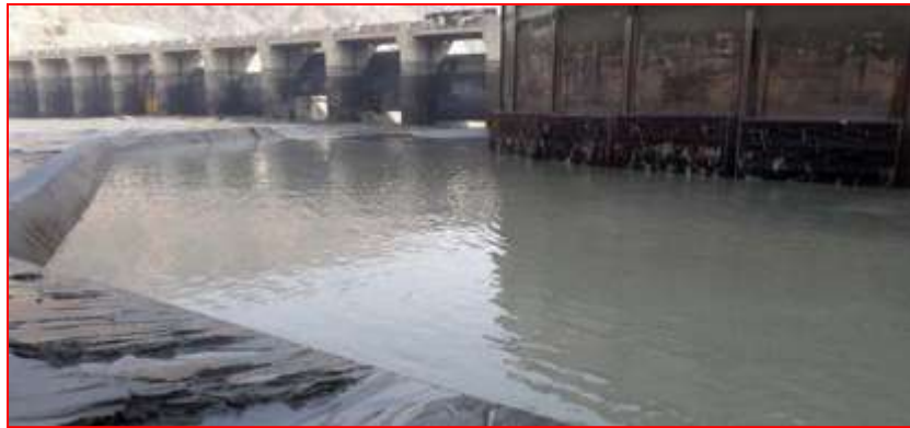
Figure 1.2: Deposited Sediments in front of Power Intake
