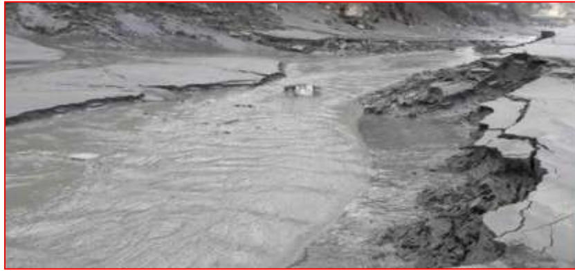
Figure 1.1: Deposited sediments in Reservoir of Warsak Dam
