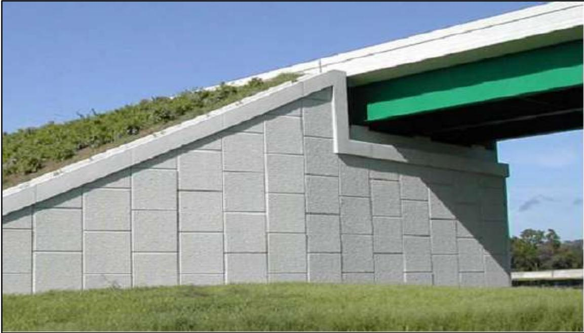
Figure 3. Bridge Abutments
