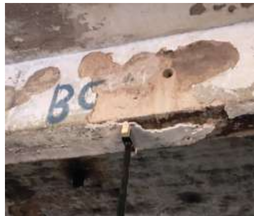
Fig. 5 Core sample from damaged beam
