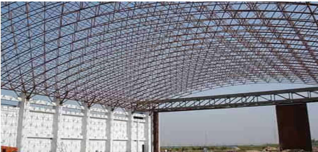
Figure-2: Large Span Space Frame
