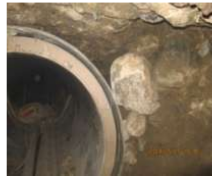
Figure 13: Interaction of pipe and boulder alongside the pipe
