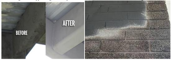
Fig (1) shoes a comparison between surfaces before and after sandblasting.
