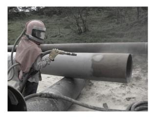
Fig (2) shows a person carrying out sandblasting
