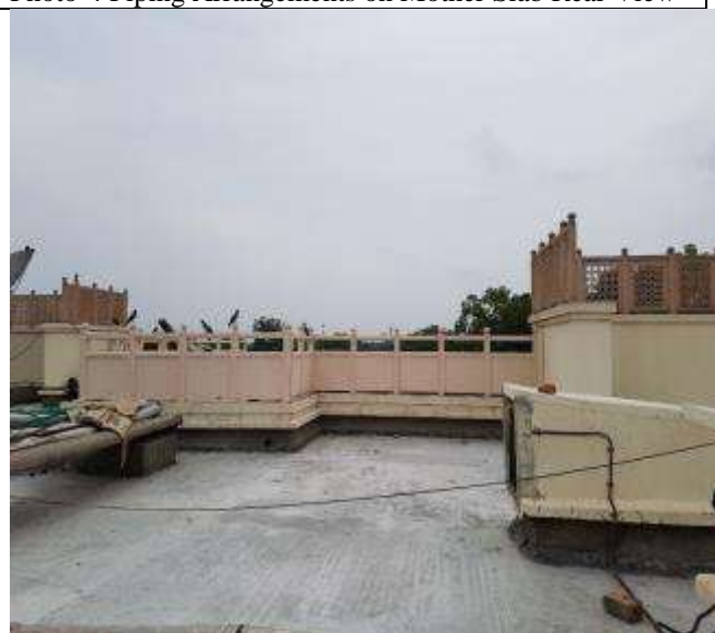
Photo-6 Another View of on Mother Slab at Point No 05
