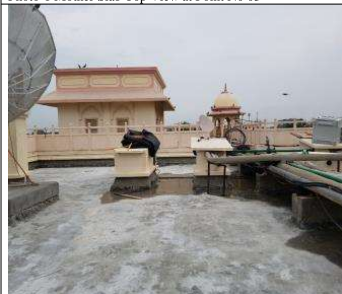
Photo- Equipment & Ducts on Mother Slab at Point No 12
