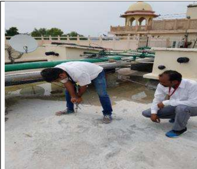
Photo-7 Rebound Hammer Testing at Mother Slab
