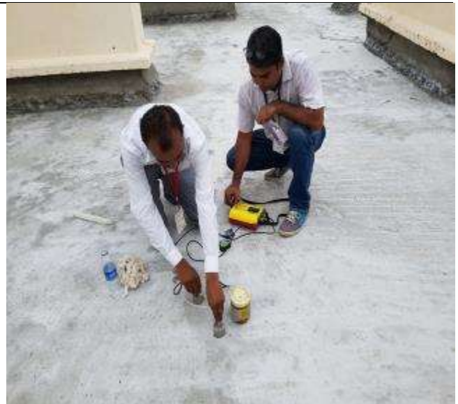
Photo-9 UPV Testing at Mother Slab
