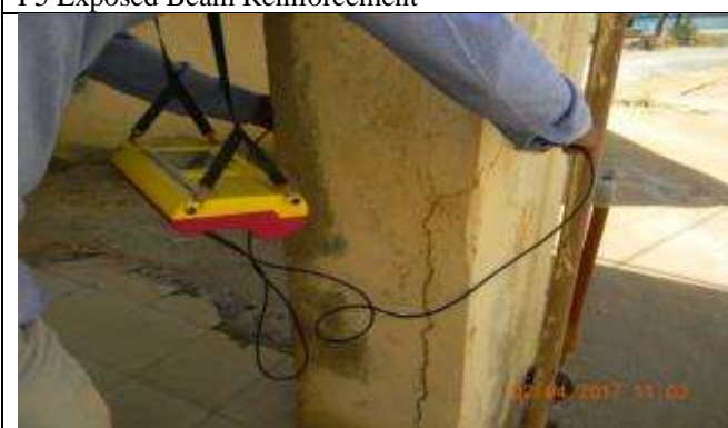
P7 Direct UPV test on Column
