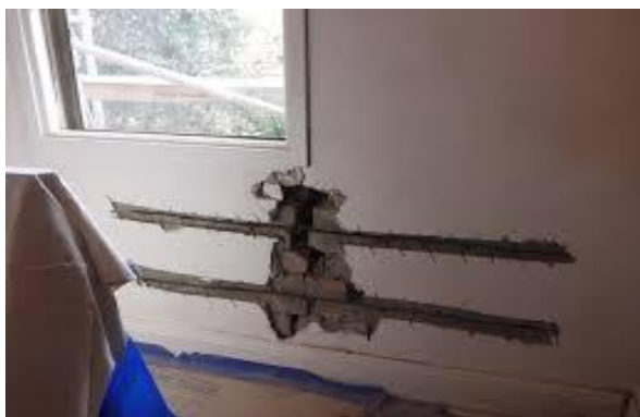
Fig No.07 Wall Cracks Stitching
