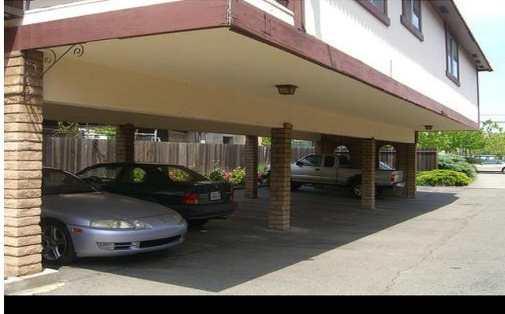
Figure 1: Ground storey of RC building are left open for parking
