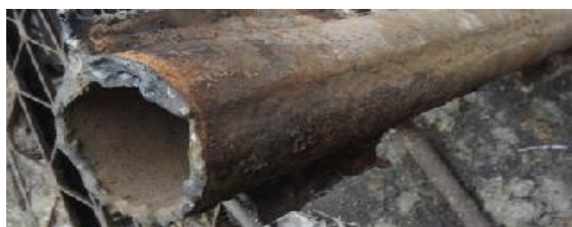
Figure 1. Thickness Reduction due to fly ash Boiler-III SGP NFL Naya Nangal.[1]
