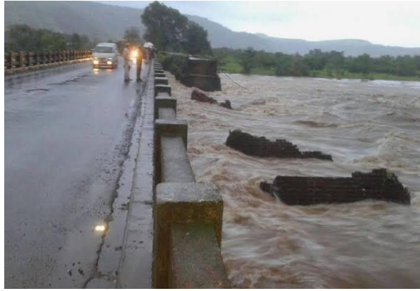
Photo 2 Failure of British era Mumbai- Goa Bridge
