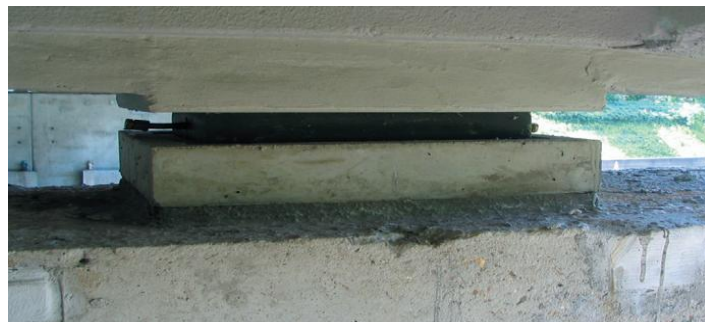
Photo 5 Bearings with anchor plates
