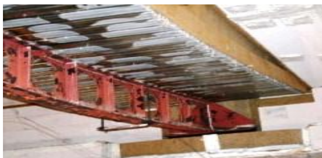
Fig 1. Flexure Buckling of Castellated Beam
