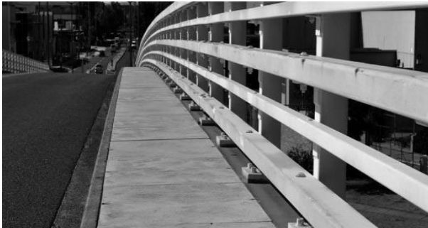
Fig.5-Salmon Street Bridge Precast Footway Panels
