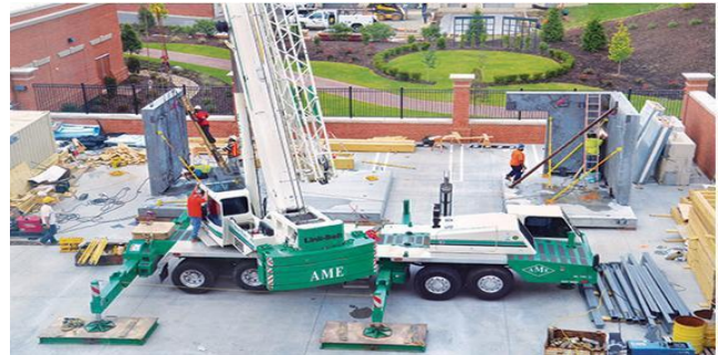
Fig.6-Geopolymer Fly Ash Concrete Walls being assembled
