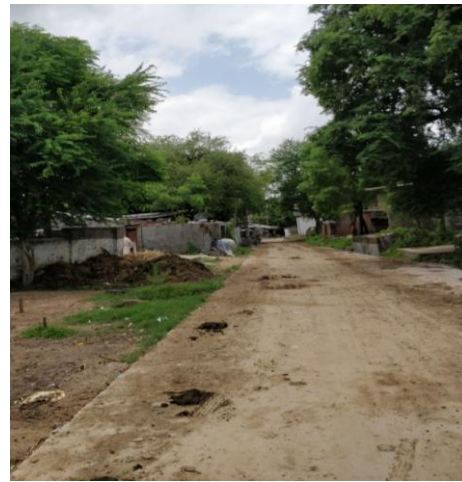
Fig - current road condition(RCC)
