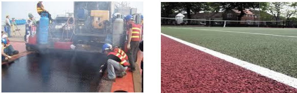
Figure 7. Tack coat application over the Membrane (Part-B)
