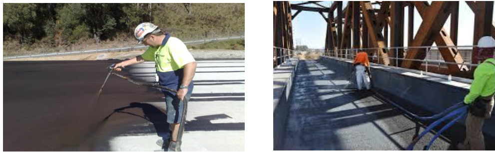
Figure 6. Tack coat application over the Membrane (Part-B)
