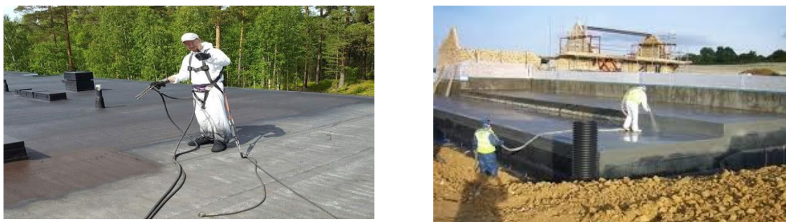
Figure 3. Application of Primer
