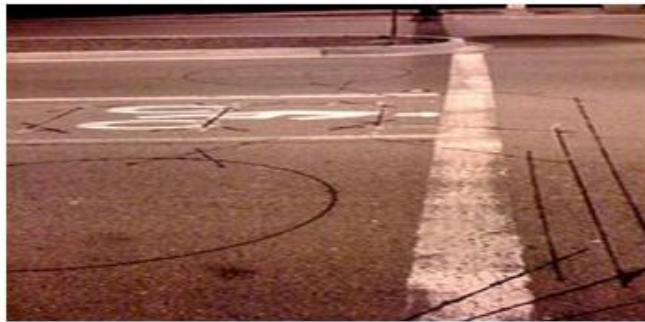
Figure 1. Electronic Circuits built into the road
