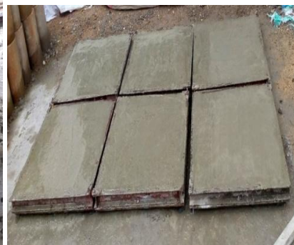
Plate 5: Casting of slab
