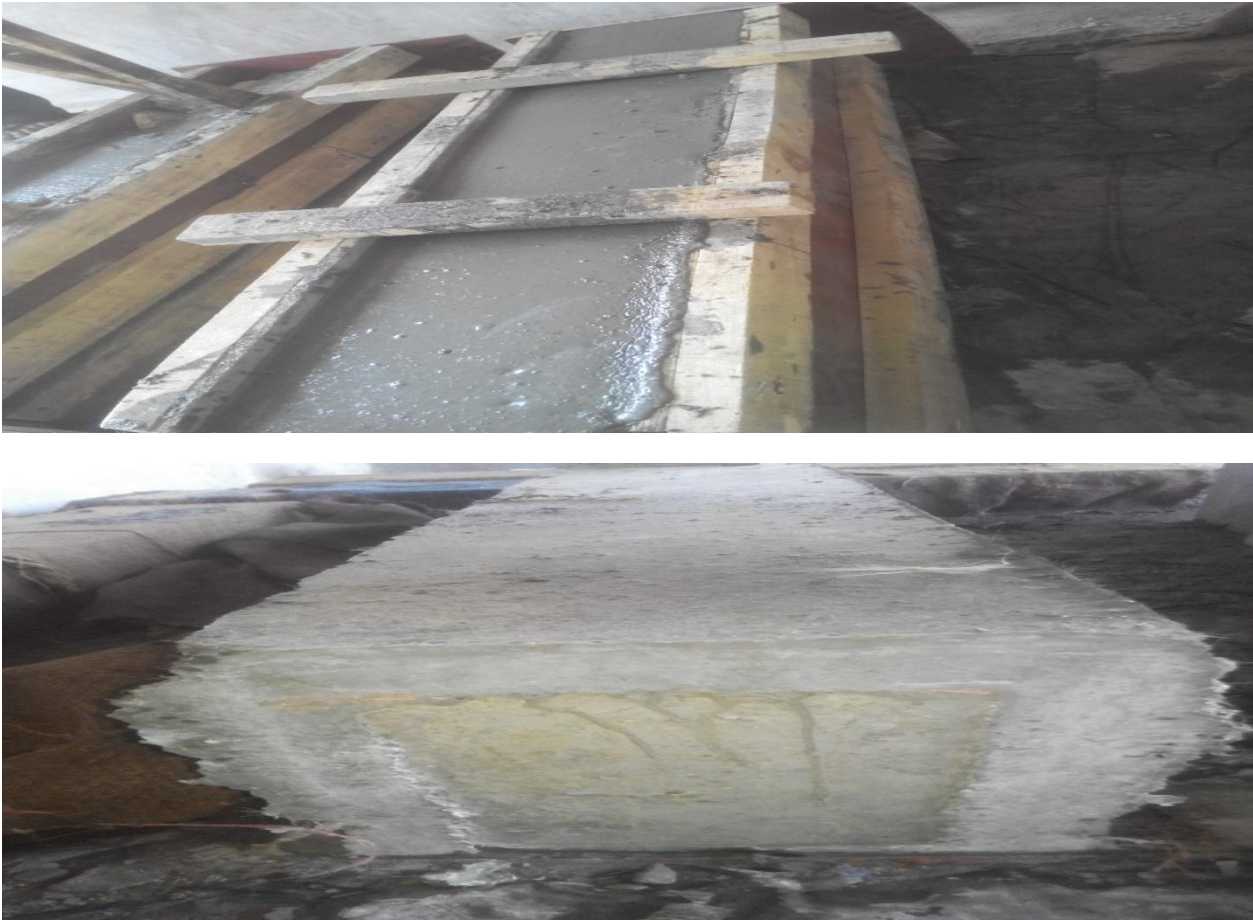
Fig .5 placing of material and final geometry of the beam after the layering
