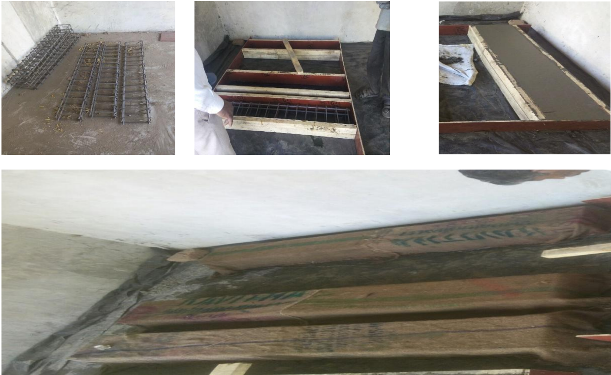
Fig.3 a) reinforcement b) formwork with cage c) concrete beam d) curing of concrete
