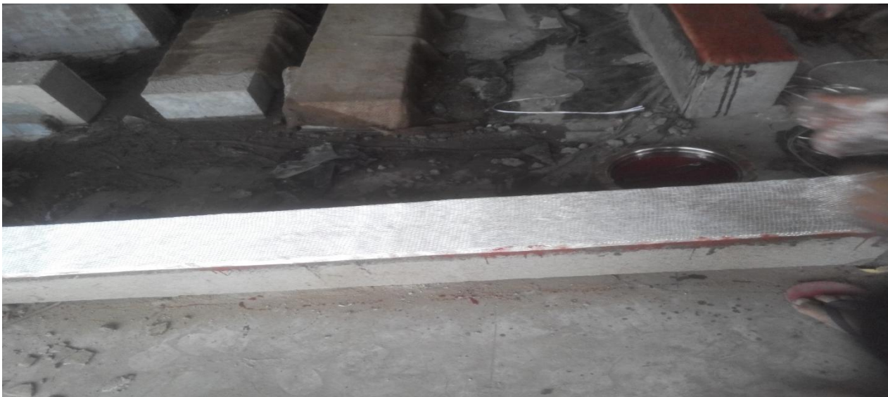
Fig. 4 After application of the primer and saturant, GFRP sheet .
